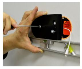
Step 2 ! Optional: The mounting plate provides an additional mounting hole on the left side. It is located outside the box directly on the wall and gives free additional stability if necessary.
